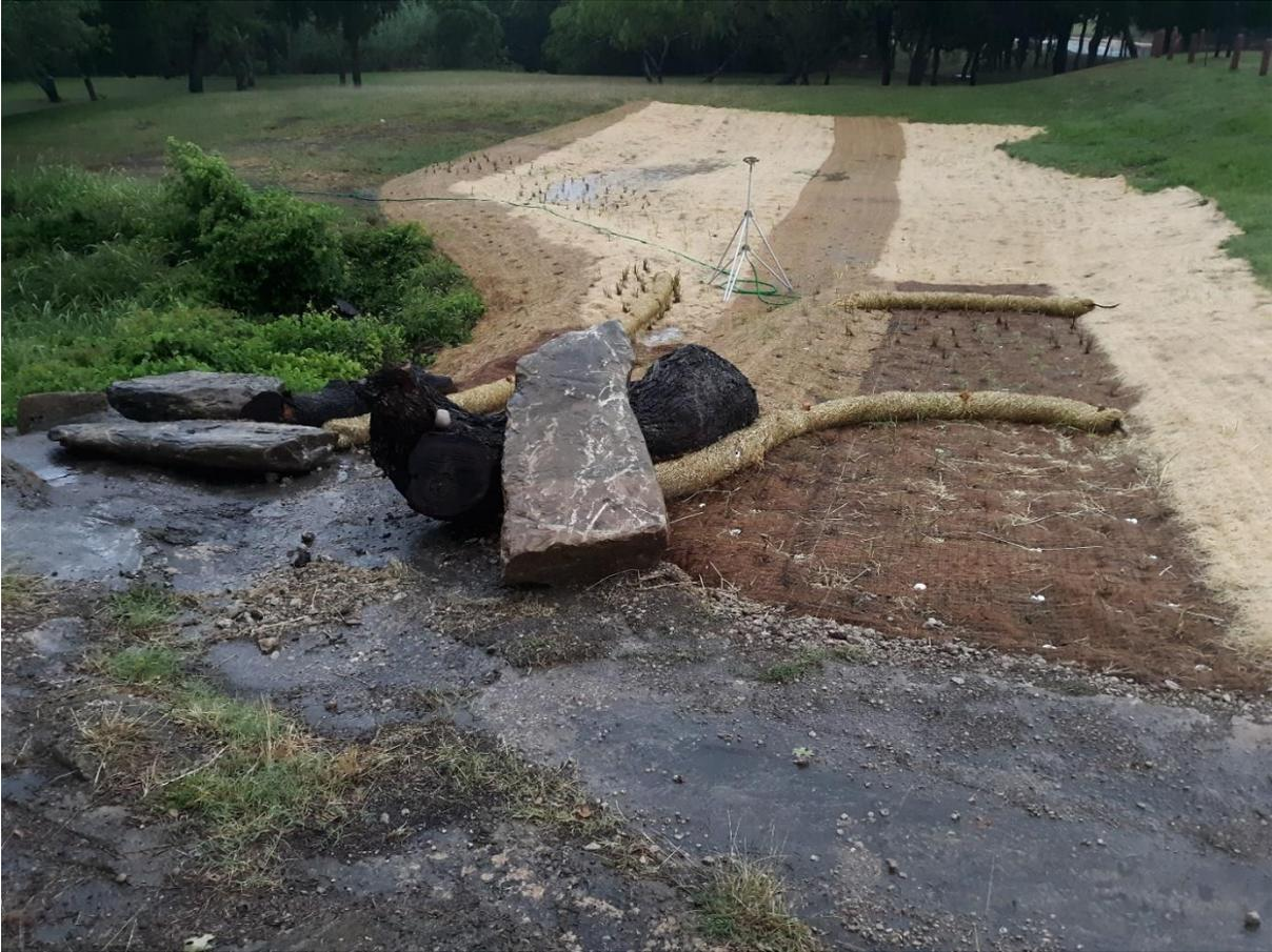
*Fig 6. Rain garden diversion point as built.*
