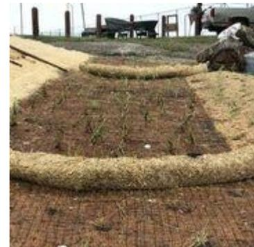
*Fig 4. A form of turf matting was installed, and riparian plants were plugged into the fabric.*
